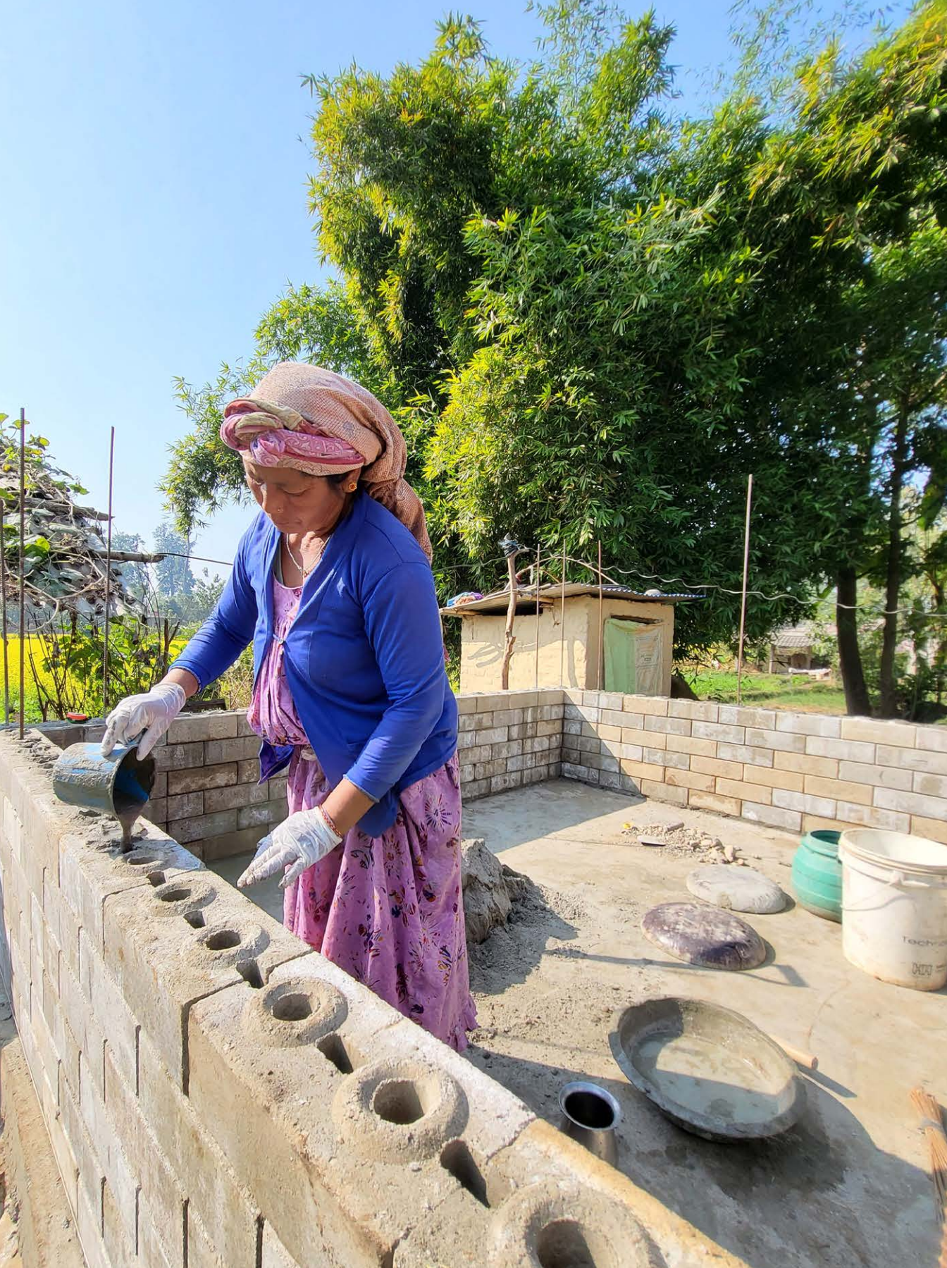
A woman builder in the process of building affordable and earthquake resistant house using Compressed Stabilized Earthen Bricks (CSEB) interlocking bricks in Kailaki district.
